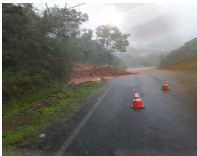
Figure 13a: Landslide along Queens after Nakorovou on the 18 th December. Source: Fiji Roads Authority
