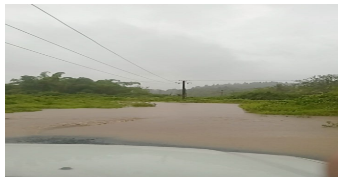
Figure 12d: Waivunu Road closed to all traffic due to flash flooding on the 18 th December. Source: Fiji Roads Authority
